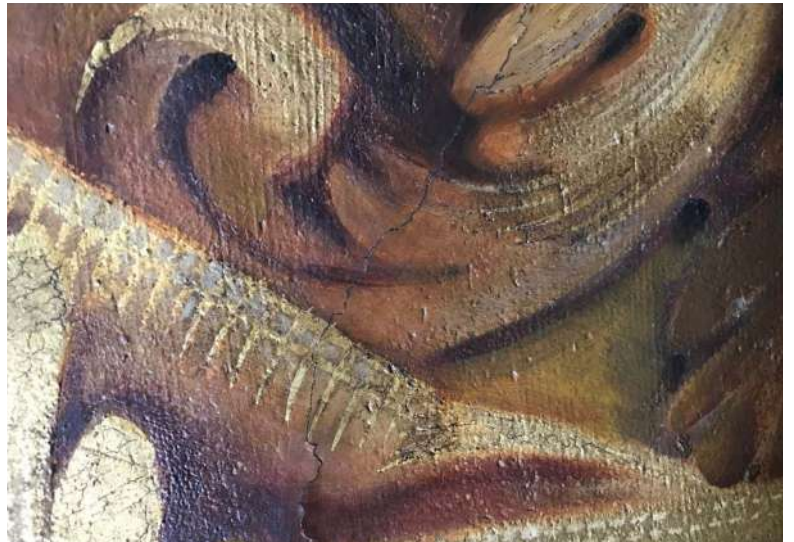
A section of the south-west platband. Re-opened crack and gaps in the mastic. © Marie Bégué
