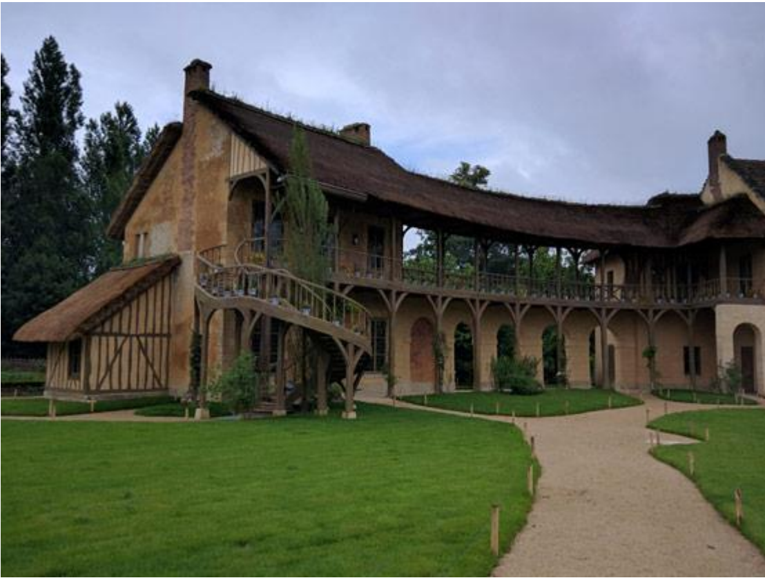
Multiple craftspeople, sponsored by Dior, restored the Hameau, which opened to the public in May 2018.
